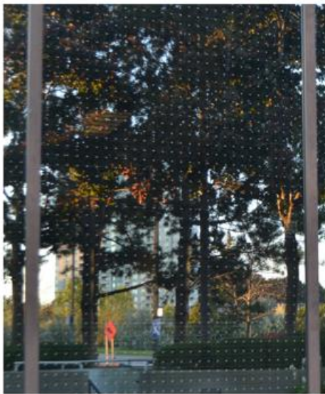
The lower level glazing of this Markham public building was treated with a 5 cm x 5 cm dot pattern, to dramatically reduce bird collisions.
