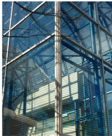
This Markham atrium was successfully treated with a "stripe", dramatically reducing bird collisions with the glass.
